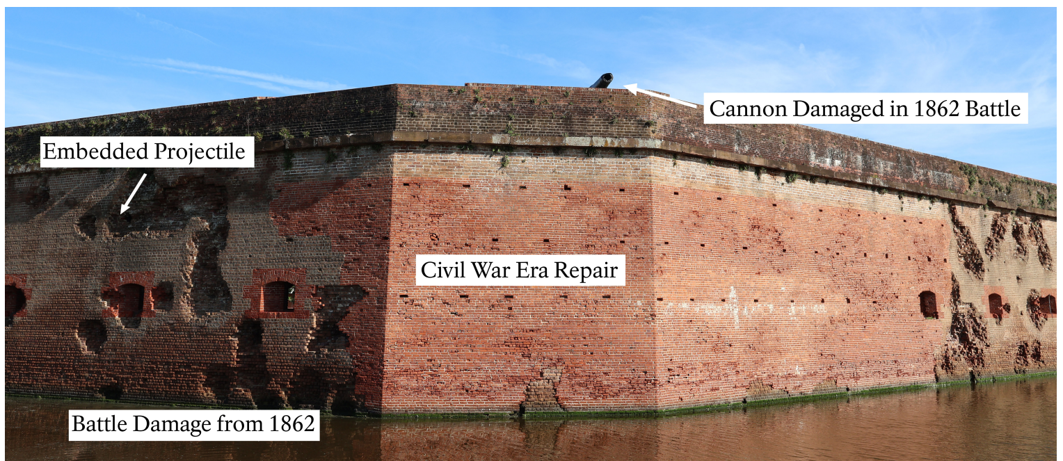
The Breached Corner was repaired during the Civil War. Battle scars still remain.
